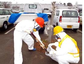
Workers removing surface soil, dust, and small rubble in the parking lot in front of the Main Anti-Earthquake Building at Fukushima Daiichi Nuclear Power Station to reduce radiation dose.
