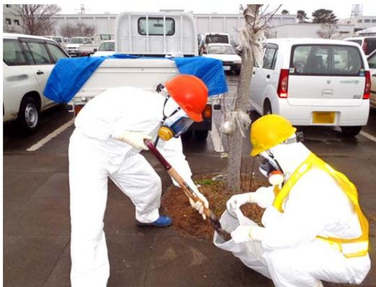
**Workers removing surface soil, dust, and small rubble in the parking lot in front of the Main Anti-Earthquake Building at Fukushima Daiichi Nuclear Power Station to reduce radiation dose.**
